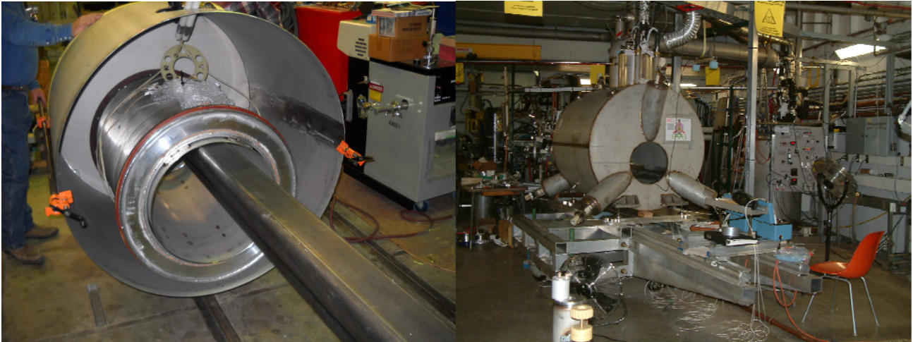
FIG. 5. Left: The original superconducting bobbin fit into its new cryostat. Right: Final assembly of Big Sol positioned back in its original location in cave 2 and reconnected with its original cryogenics and power supply systems.
