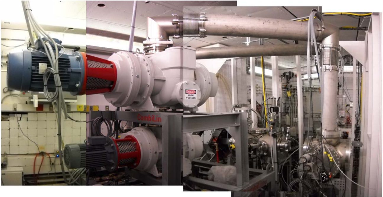
FIG. 9. The tubes connecting the 3x tier roots blower system to the light ion guide chamber have been installed and the Light Ion Guide HV platform was tested up to 8 KV.
